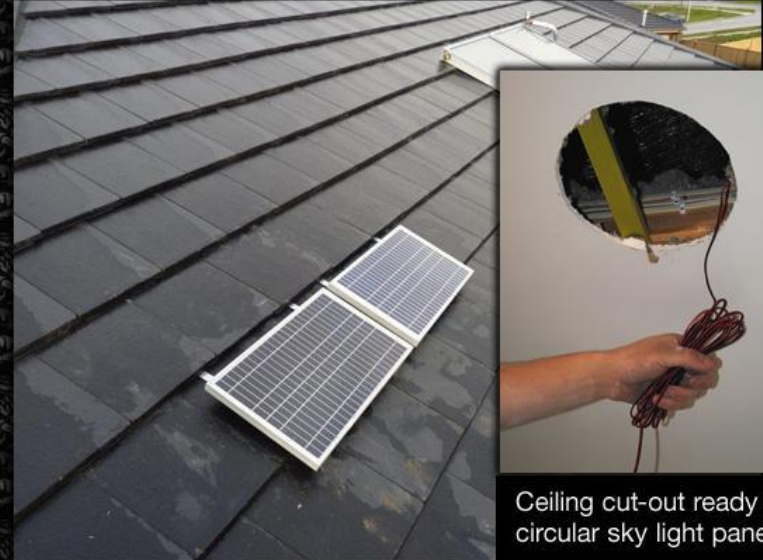
Two Solar Collectors installed to a tiled roof
